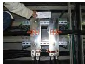
↑ supporting plate with slight movement.
