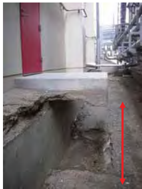
← Entrance for the Hall. About 1 m gap.
