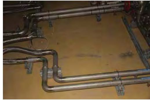
Crack observed on March 28 after pumping water. 3
