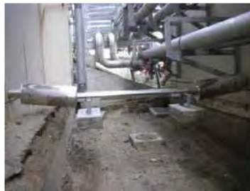
↑ Disconnected pipes Distortion of bellows →
