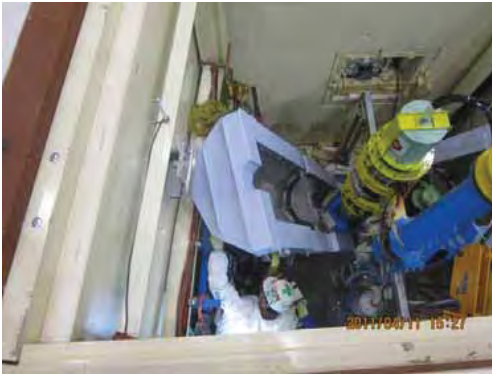
↑ Removal of Pb shield wall.
