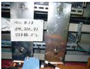
↑ supporting plate with slight movement.
