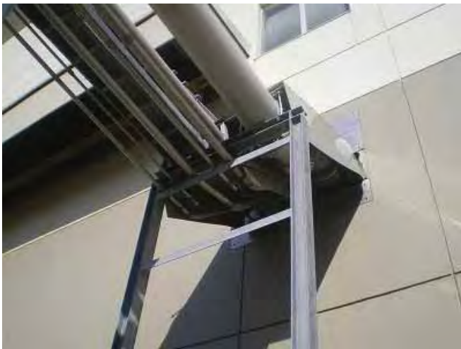
Sinking caused a sharp bend in the piping system though the building (upper).
