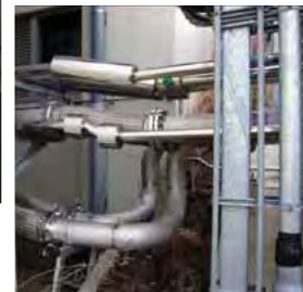
↑ Disconnected pipes Distortion of bellows →
