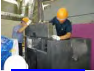
Lead shield assembling
