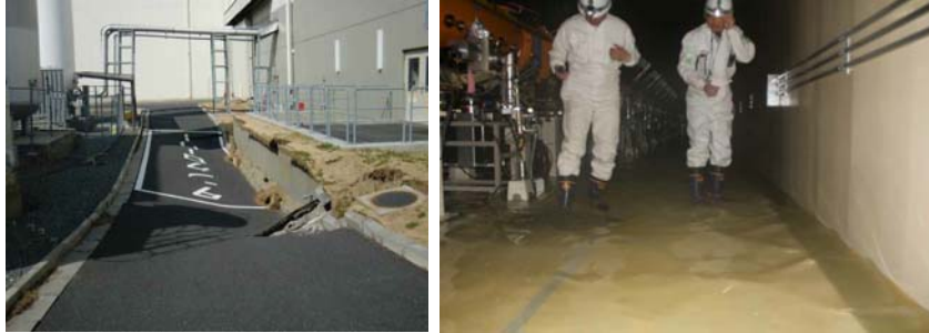
West side road from MLF. About 1.5 m sinking was observed. On March 17 the water level was only 1 cm, whereas it was 10 cm on March 24. With motor driven electric generator a pumping started on March 25.
