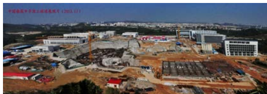
Site Civil Construction Status (Nov. 2013)
